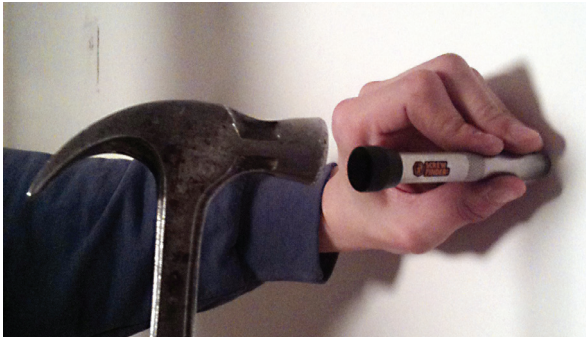
MARK LIGHTLY WITH A HAMMER WHEN SCREWFINDER FINDS THE SCREW. THE SCREW IS EXPOSED.
